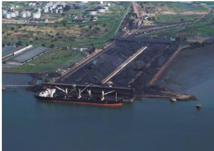
Matola dry bulk terminal, Maputo (Mozambique)
