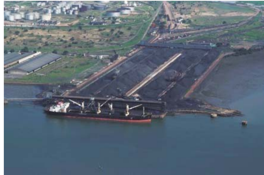
Matola Dry Bulk Terminal, Maputo (Mozambique)
