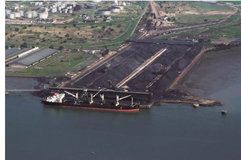
Matola Dry Bulk Terminal
