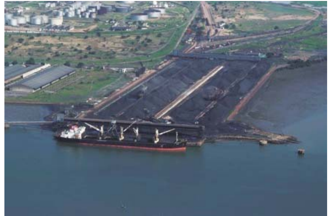
Matola dry bulk terminal, Maputo (Mozambique)
