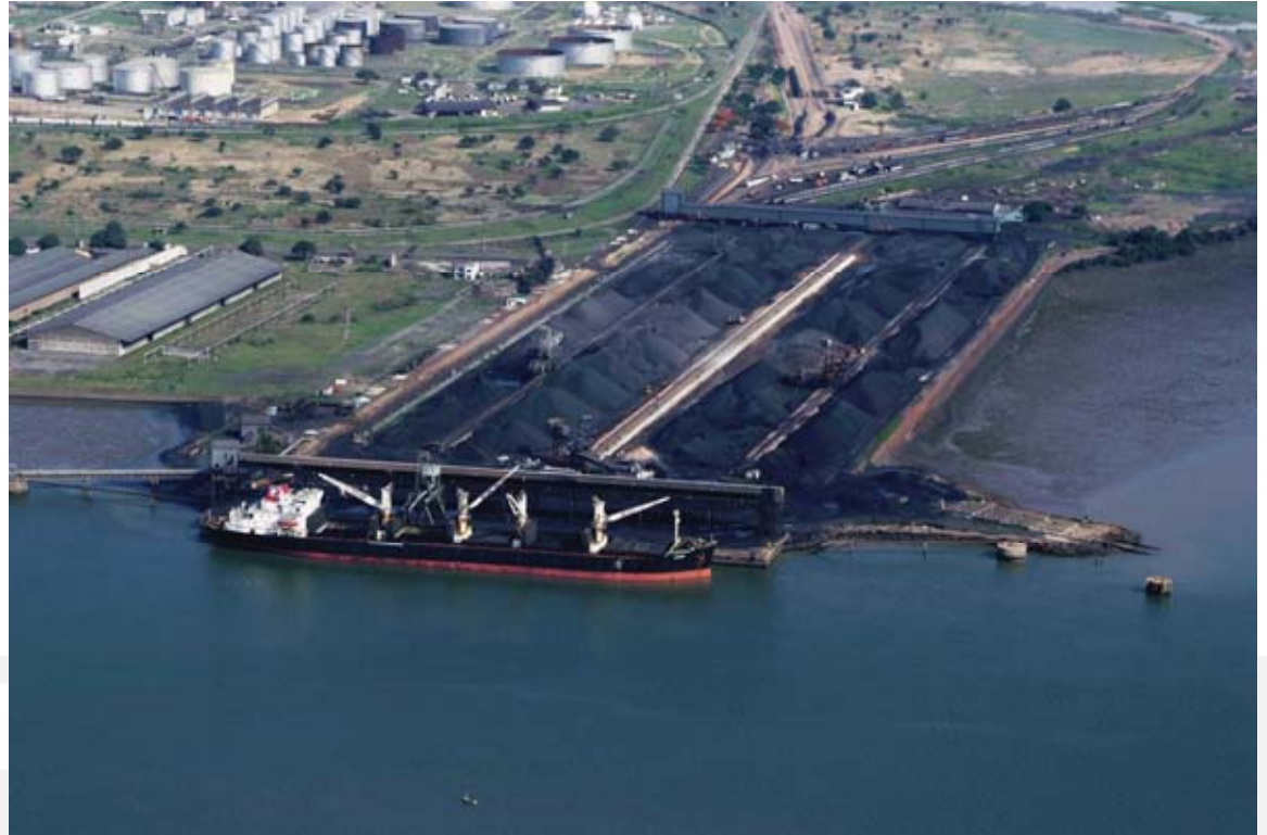
Matola dry bulk terminal
