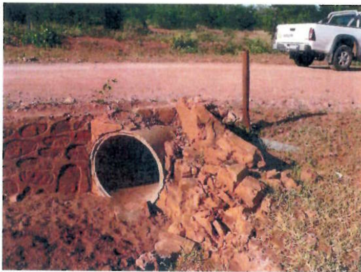
Figure 6: Broken wing walls and pipe culverts
