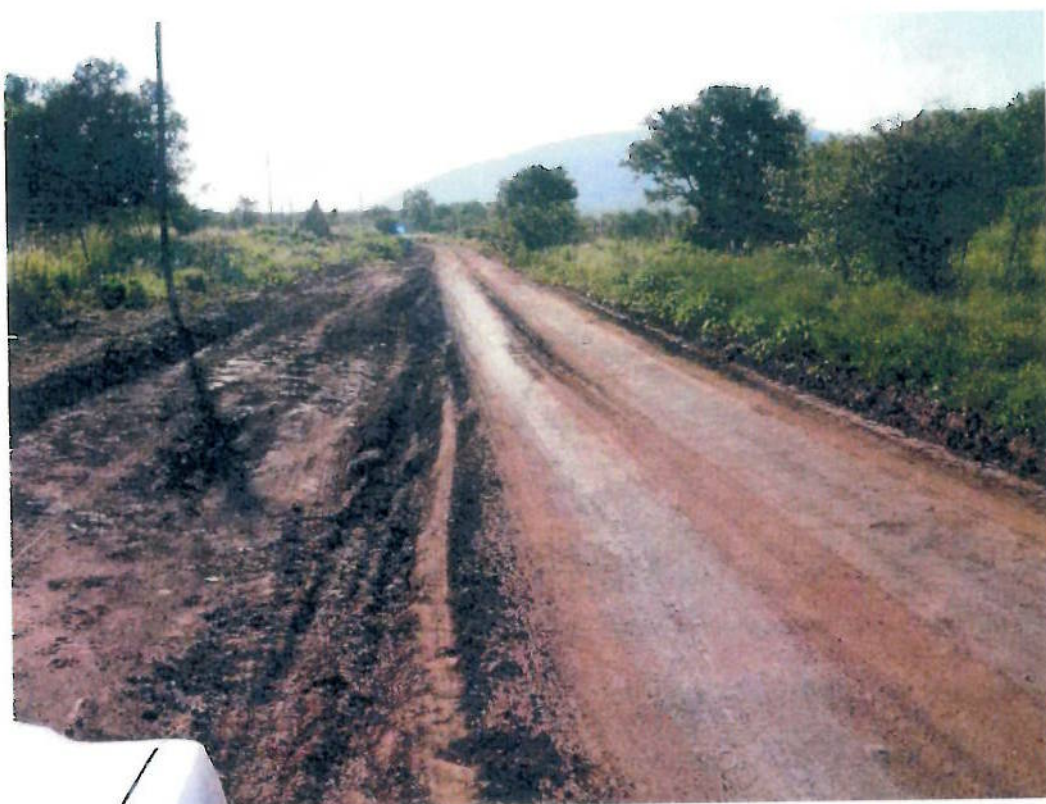
Figure 4: Makushu Road east of Mutamba Bridge crossing
