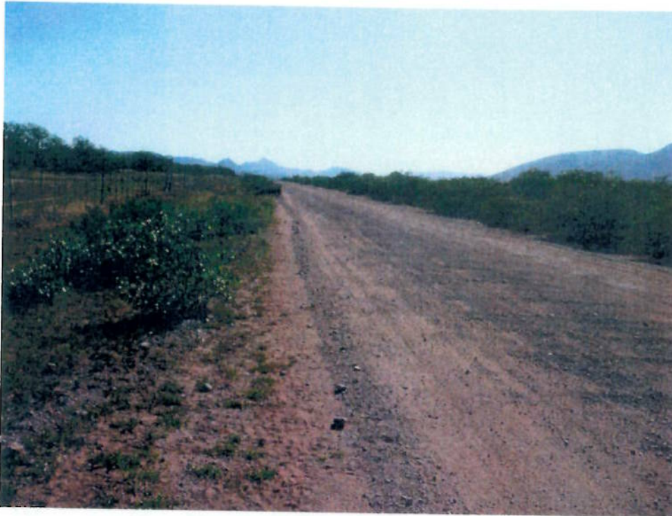
Figure 2: Nzhelele Road surface showing corrugations
