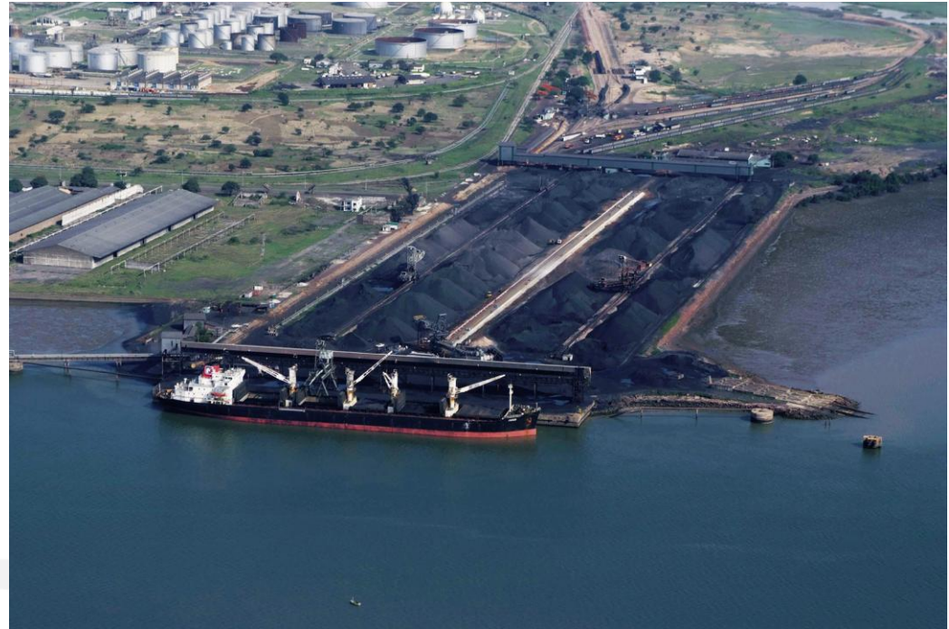
Matola dry bulk terminal
