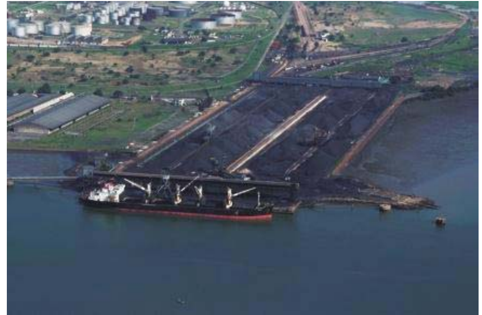
Matola Dry Bulk Terminal, Maputo (Mozambique)
