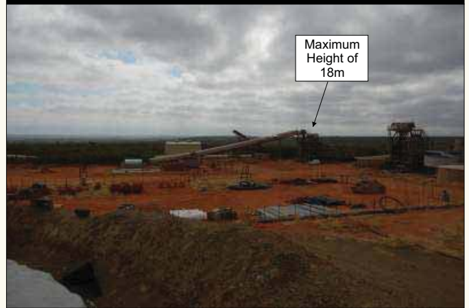
VIEW OF PLANT INFRASTRUCTURE
